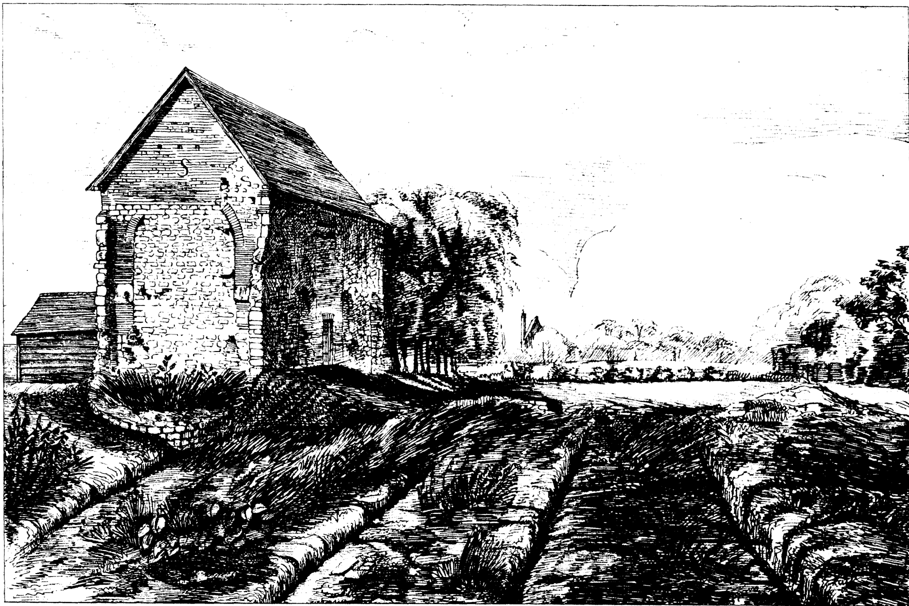
7 St Peter's church, Bradwell-on-Sea, showing the trenches excavated in 1864
