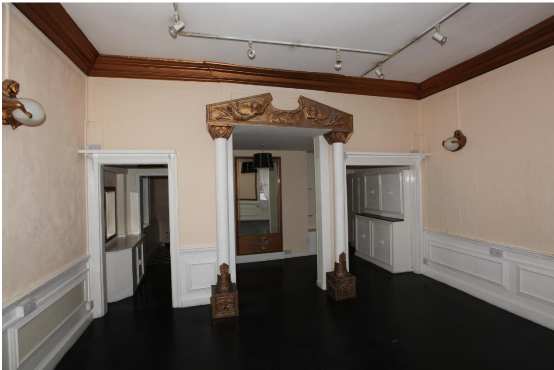
Illus. 21. The rear wall of the front room above the party shop (O). The narrow bay between the two door surrounds was designed for a chimney with back-to-back fireplaces, but sadly this was entirely removed after 1951 (figure 16 shows five chimney pots, of which one - perhaps a later addition – probably served the attic room). The cornice steps forward to respect the missing fireplace, but the broken pediment and columns are modern set dressing for a hair salon that formerly occupied the premises.
