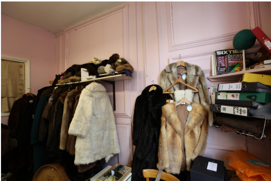
Illus. 17. The fine bolection-moulded panelling and first-floor fireplace to the west of the central chimney in the charity shop (now in the manager's office, V). The door on the right opens into the cupboard shown in illus. 16 above (W). This is the only original chimney not to have lost its external stack, although it now contains a WC on the ground floor. Panelling of this period was invariably painted and early pigment may survive beneath the modern surface.
