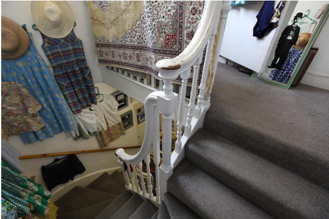
Illus. 18. The back stair in the charity shop (I/Q), with identical balusters and mouldings to the main staircase but lacking its open strings. The attic rooms are reached by a separate stair from the landing on the right. The presence of two 18 th century stairs of this quality illustrates the exceptional status of the house.
