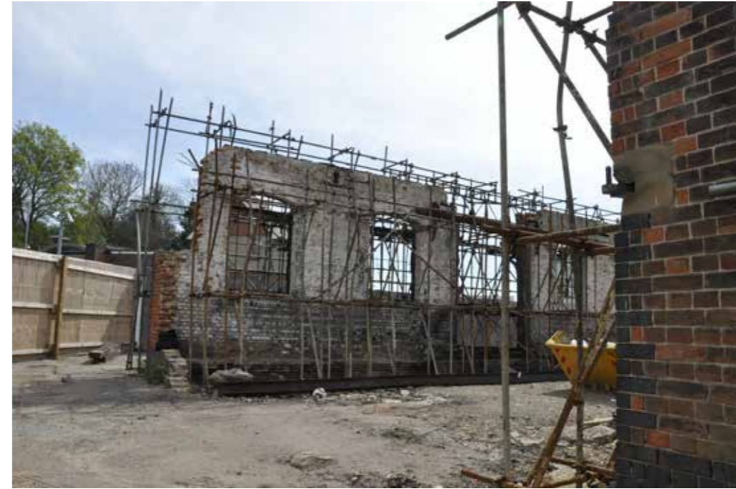
Figure 45: East interior elevation showing lack of internal features (2016)
