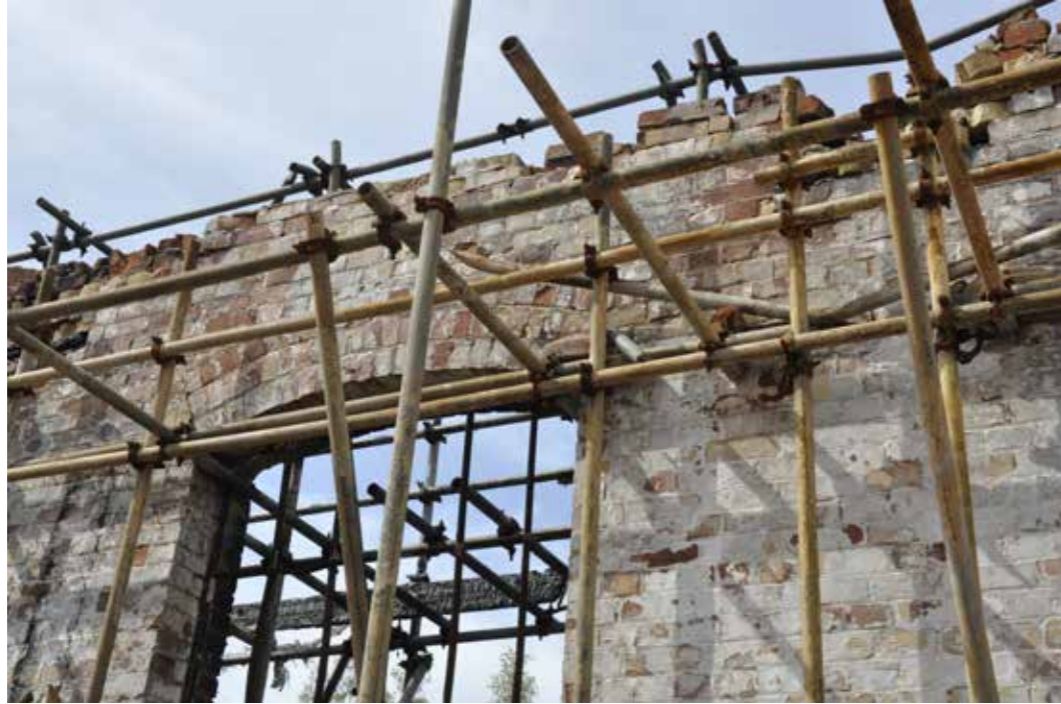
Figure 48: Close-up of damaged west interior elevation (2016)
