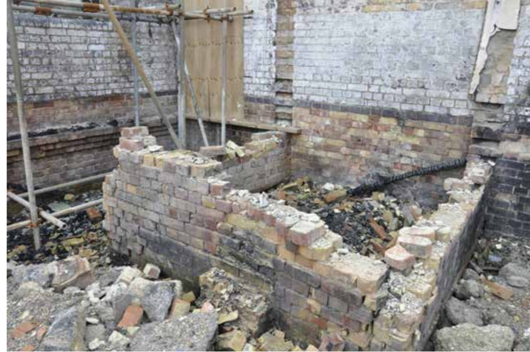
Figure 49: Detail of damaged interior platform structure (2016)
