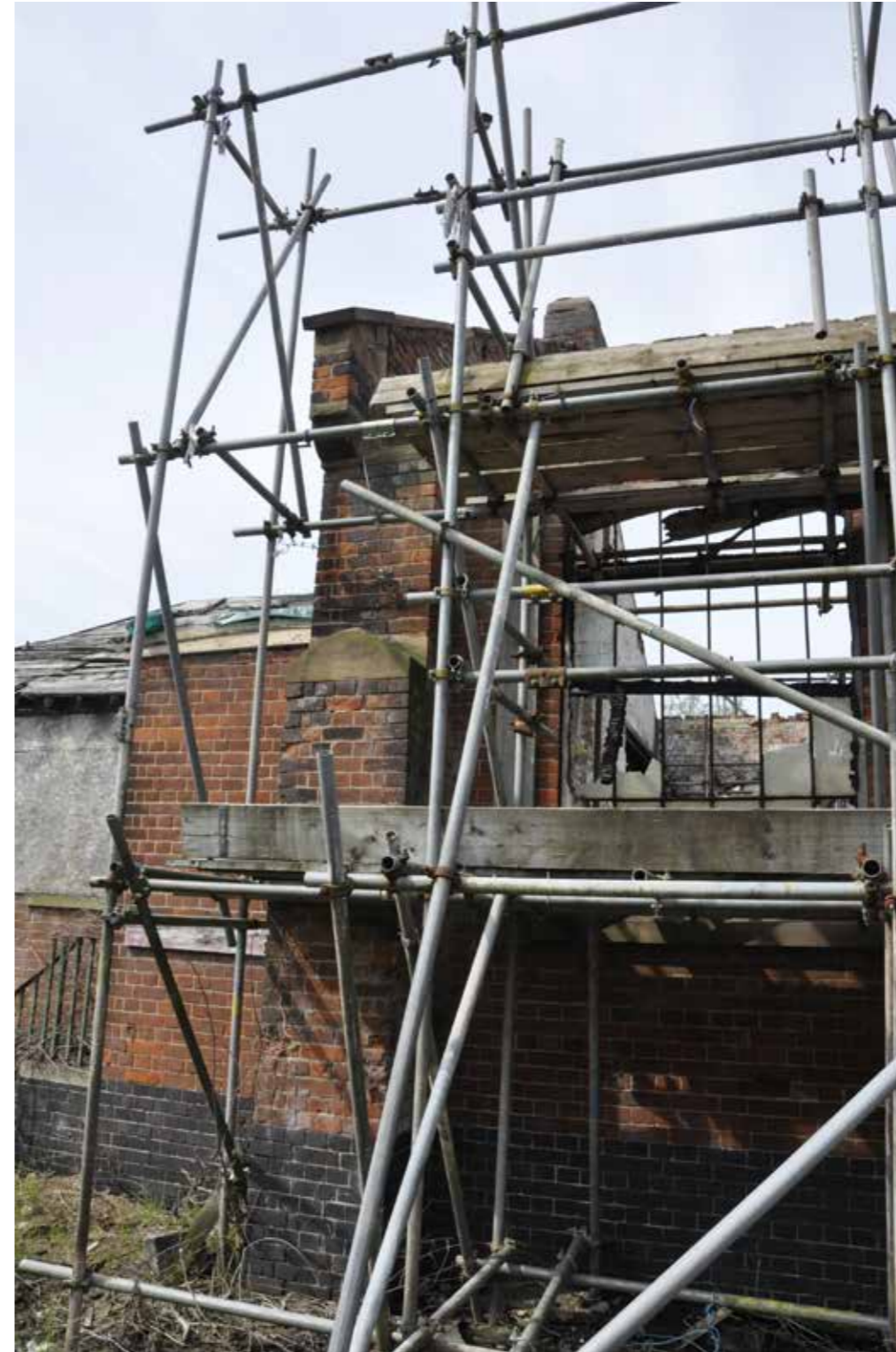
Figure 20: Detail of east elevation showing sixth bay window and loss of roof (2016)
