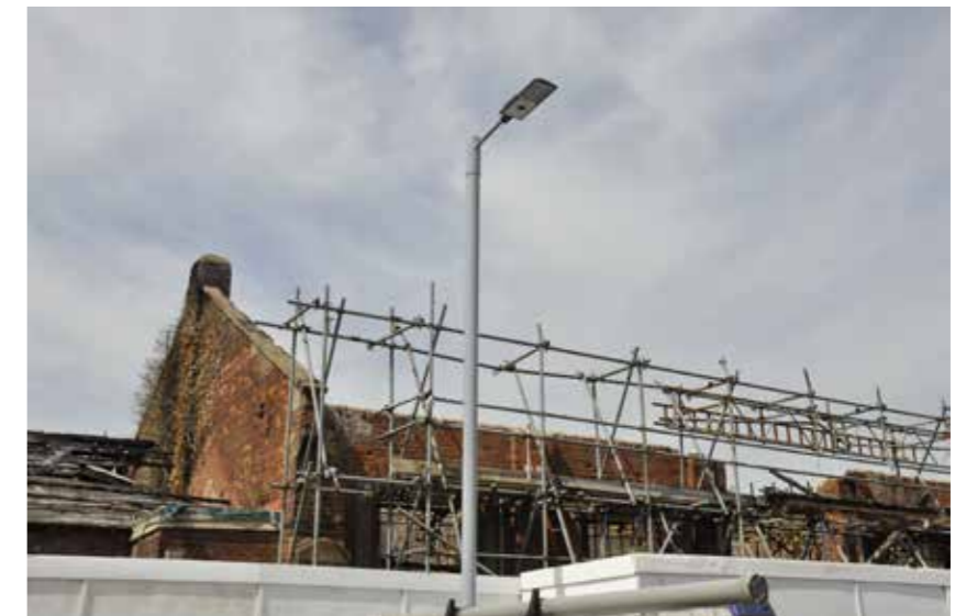
Figure 14: Former roof line seen from the station car park (2016)
