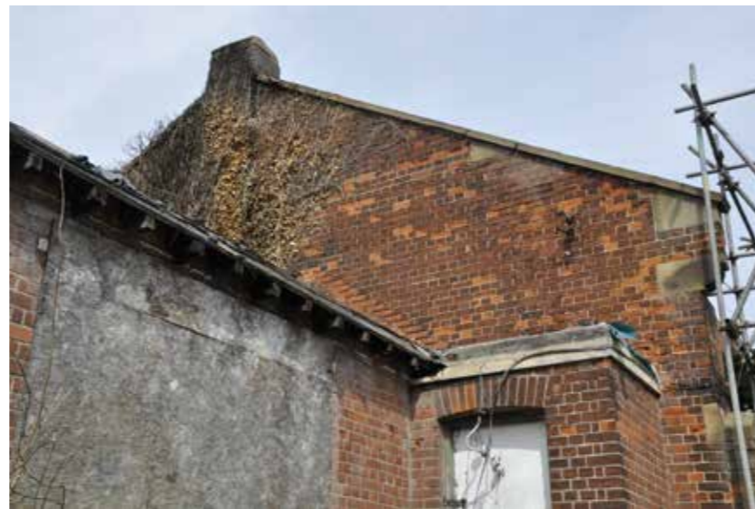
Figure 38: Detail of south east elevation (2016)
