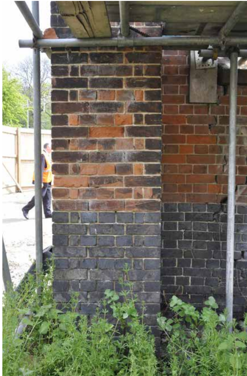
Figure 25: Detail of subsidence on west elevation (2016)
