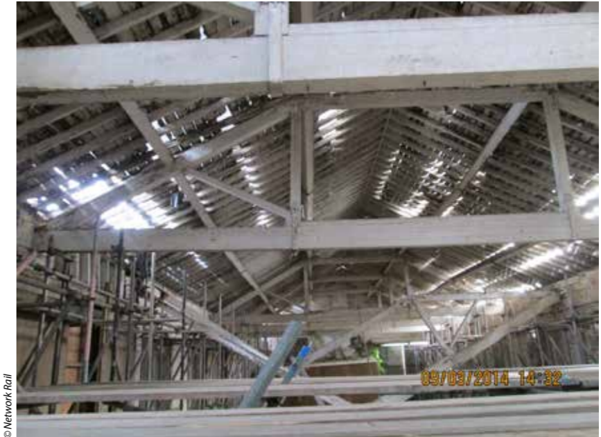
Figure 9: Wivenhoe Goods Shed roof structure in 2014
