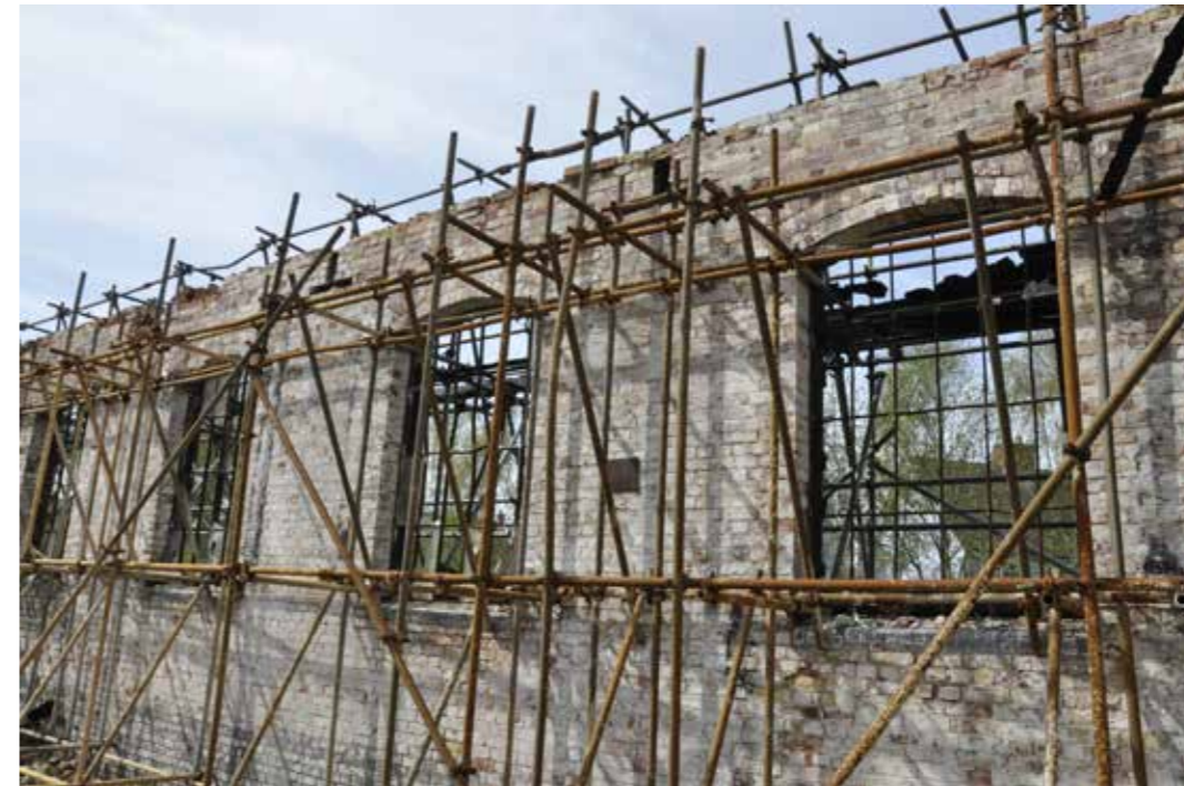
Figure 47: West interior elevation showing damaged cast-iron casements and loss of roof (2016)
