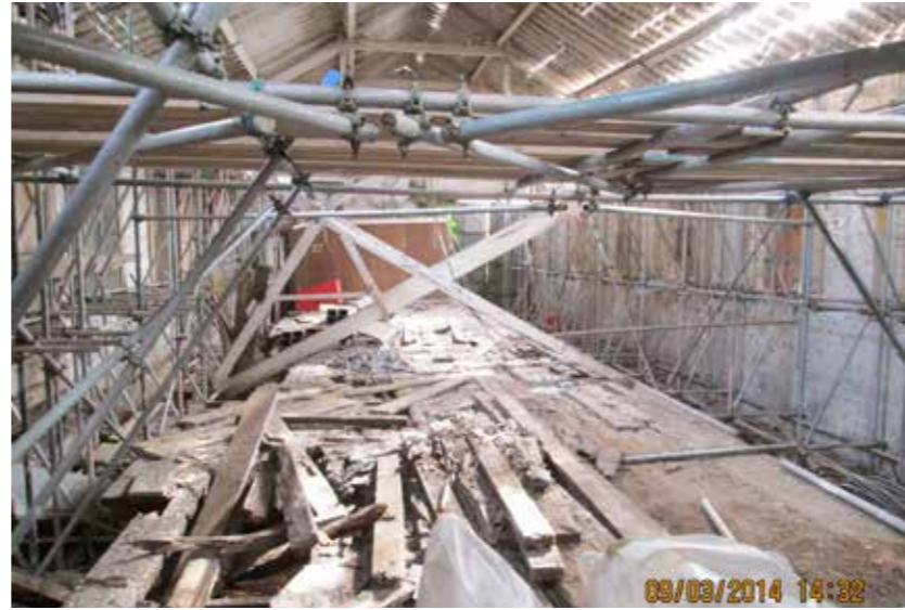
Figure 40: Goods shed platform photographed in 2014
