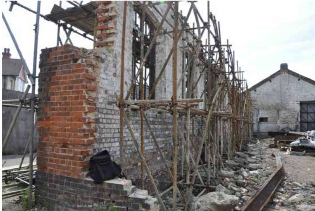
Figure 44: Close-up of east interior elevation showing lack of internal features (2016)
