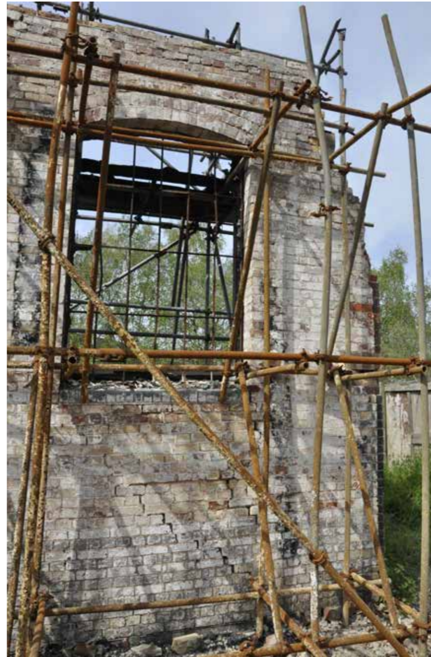
Figure 26: Detail of north-west corner showing subsidence (2016)
