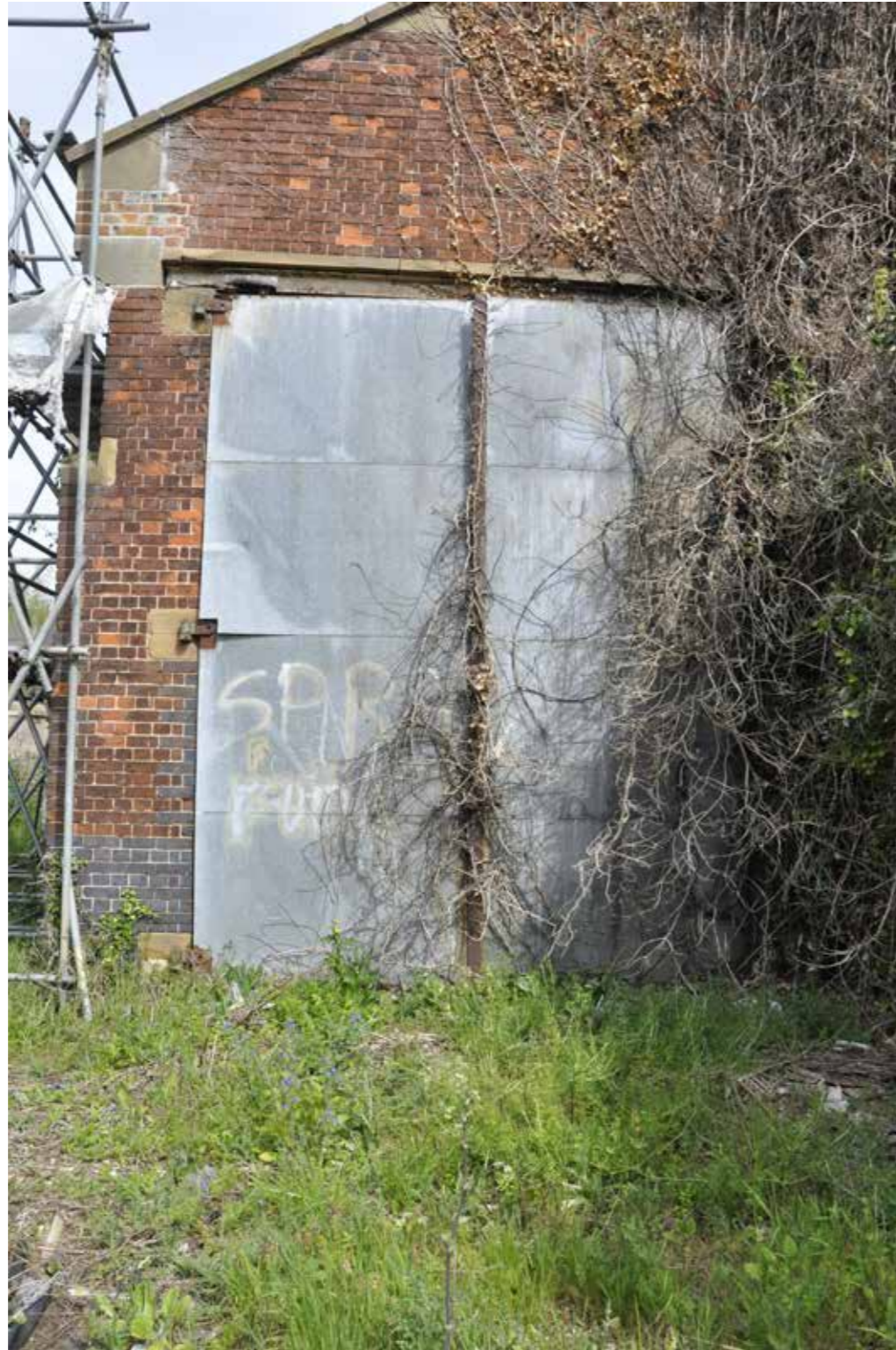
Figure 32: Steel replacement doors on south elevation (2016)
