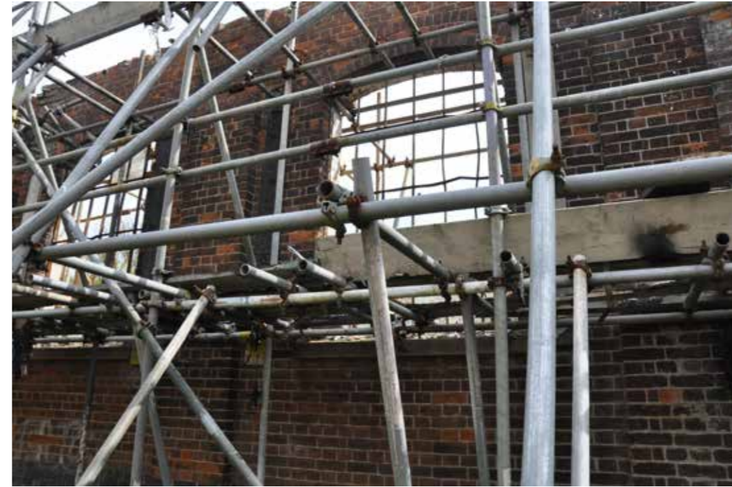
Figure 22: Detail of west elevation showing damaged cast-iron casements and loss of roof (2016)
