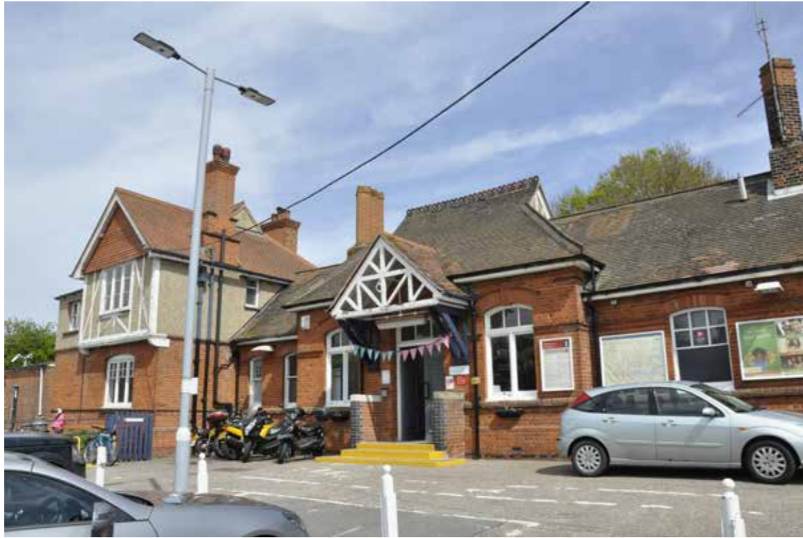
Figure 2: Wivenhoe Station rebuilt by the GER in 1886
