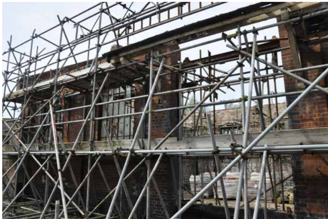
Figure 30: Detail of damaged second lean-to canopy on east elevation (2016)
