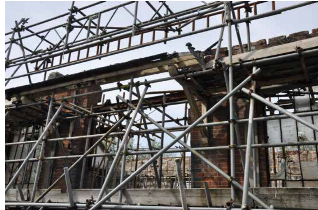
Figure 18: Detail of east elevation showing damage to second lean-to canopy and loss of roof (2016)
