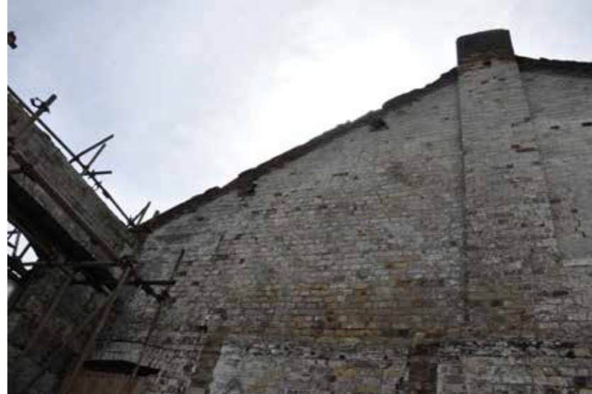
Figure 42: Detail of south elevation showing loss of roof structure (2016)
