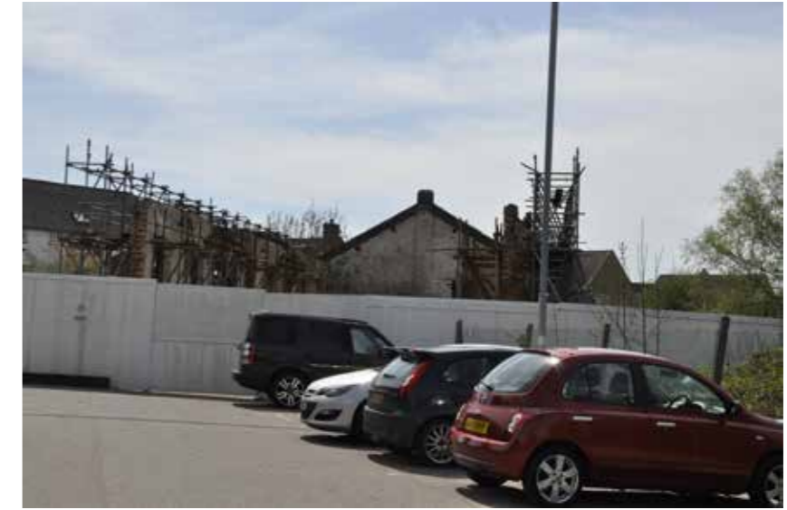
Figure 12: Exterior viewed from the north showing demolished elevation and loss of roof (2016)
