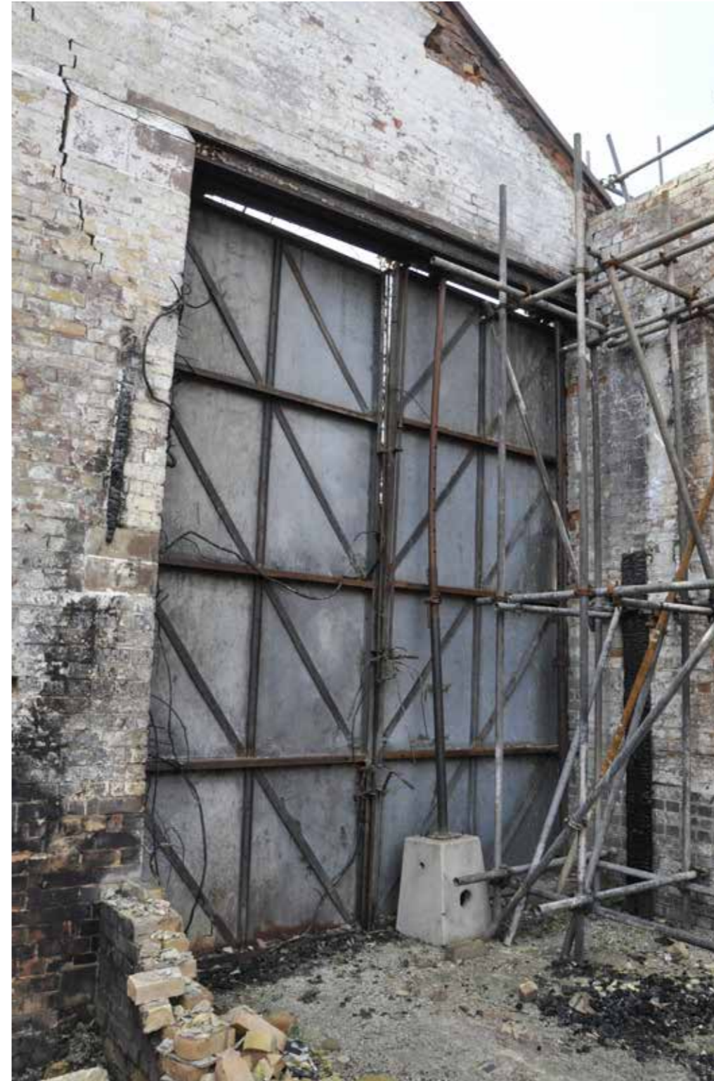
Figure 33: Steel replacement doors on south elevation seen from interior (2016)
