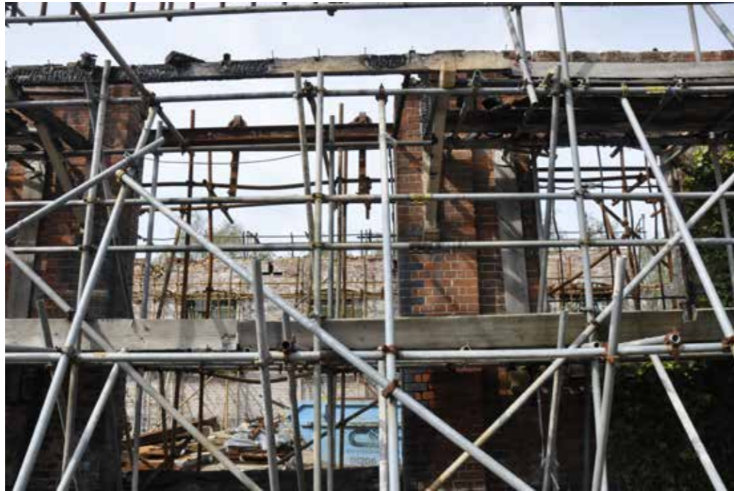
Figure 28: Detail of damaged first lean-to canopy on east elevation (2016)
