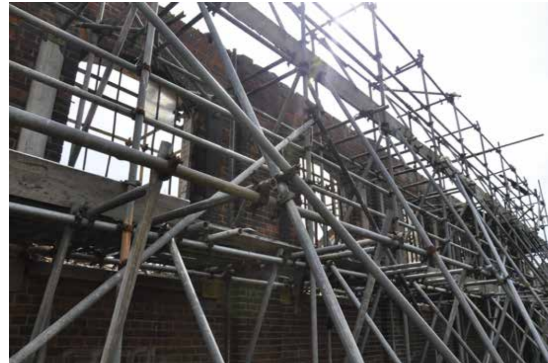
Figure 24: West elevation under scaffolding (2016)
