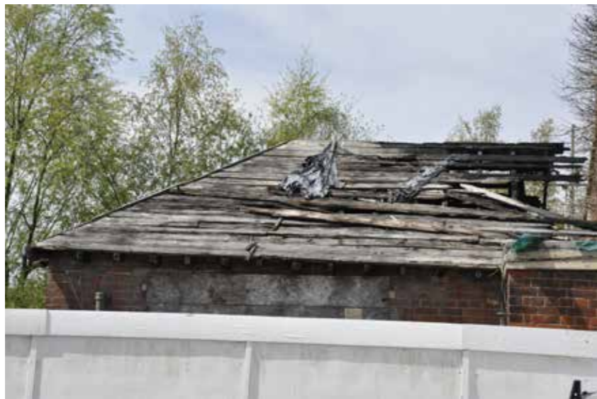
Figure 37: Small office building details of roof on east elevation (2016)
