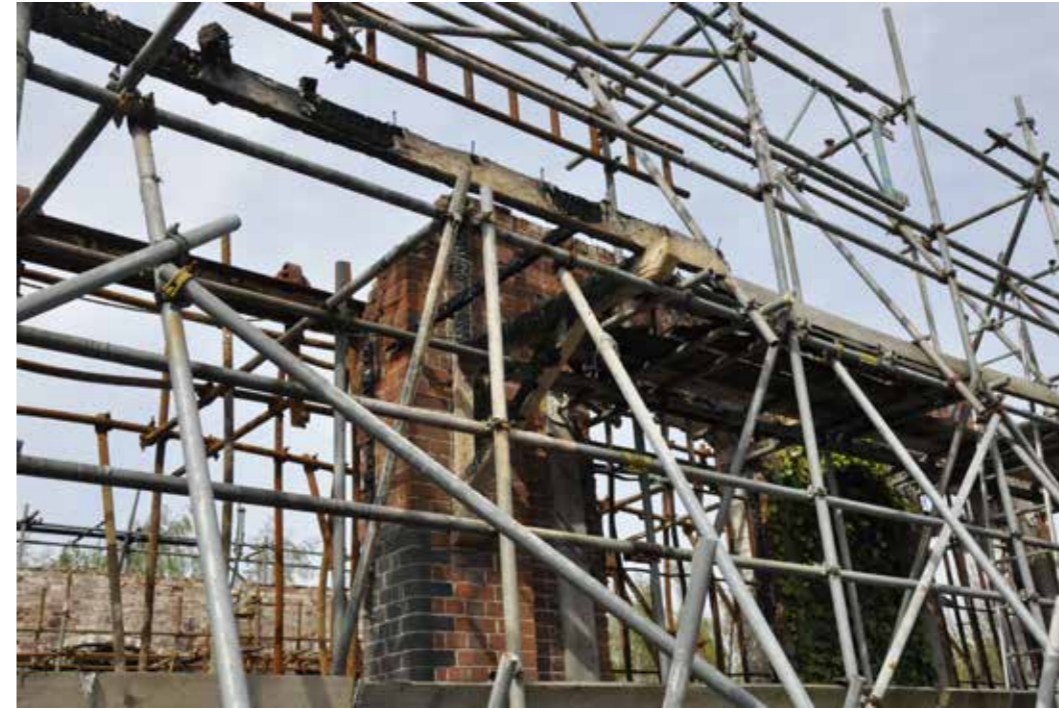
Figure 29: Close-up detail of former roof structure to first lean-to canopy on east elevation (2016)
