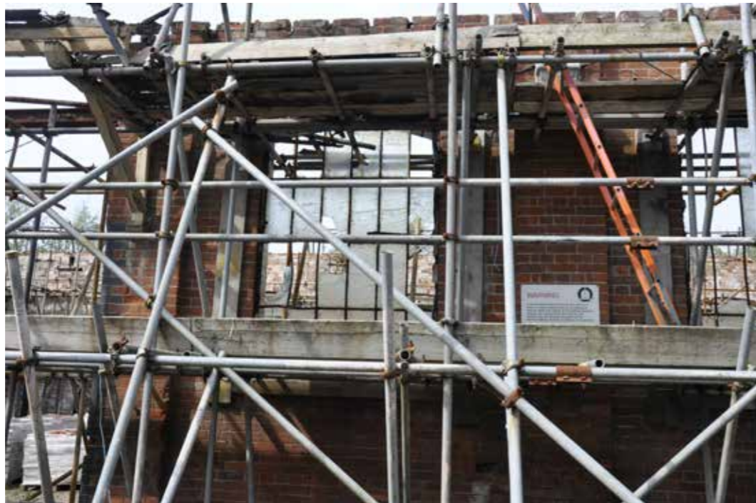
Figure 17: Detail of east elevation showing damaged cast-iron casements (2016)
