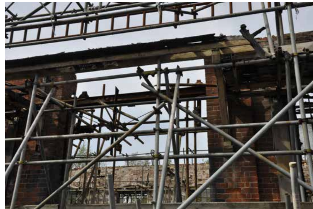
Figure 31: Close-up detail of former roof structure to second lean-to canopy on east elevation (2016)
