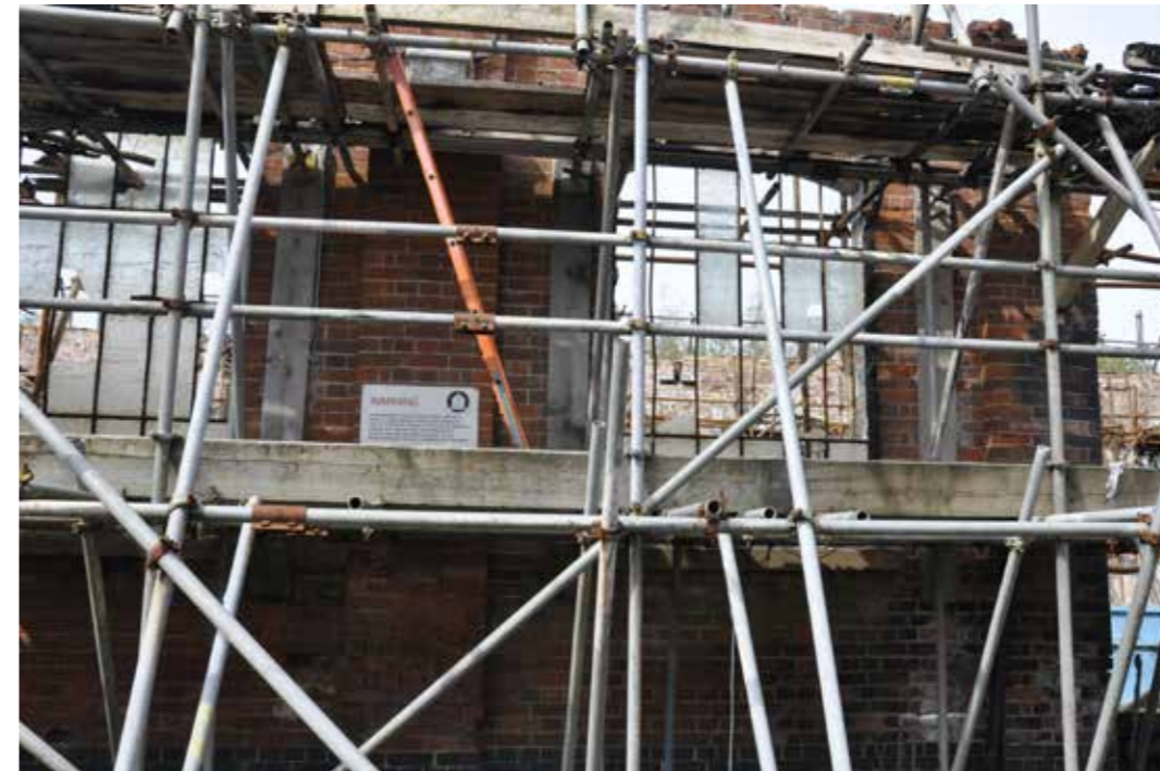
Figure 16: Detail of east elevation showing detail of damaged cast-iron casements (2016)
