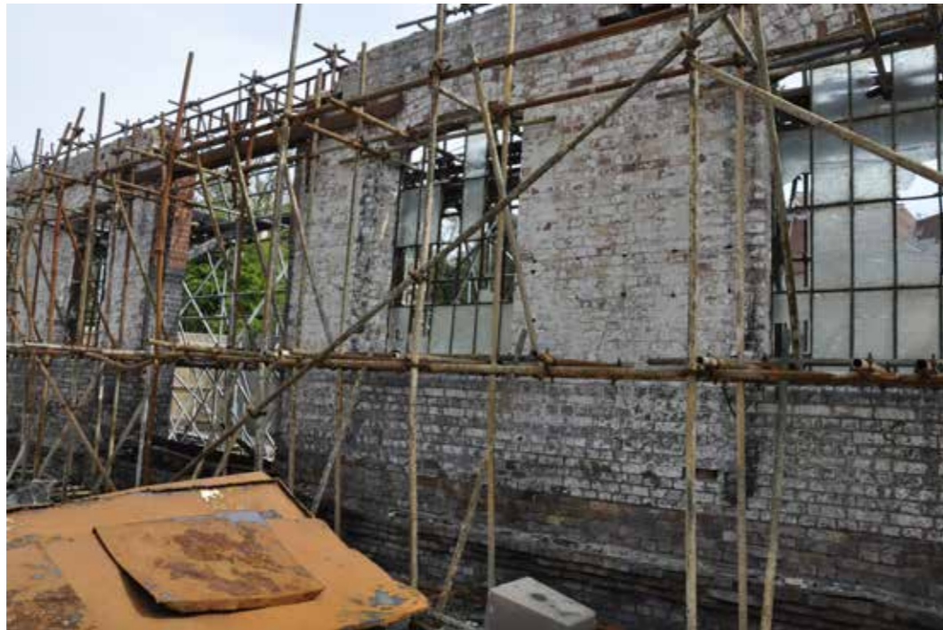
Figure 46: Close-up of east interior elevation showing lack of internal features (2016)
