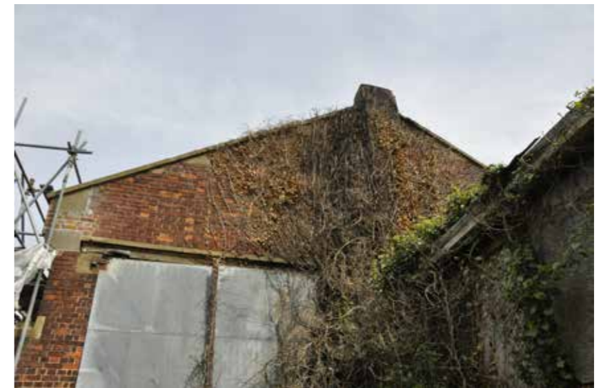
Figure 39: Detail of south west elevation (2016)
