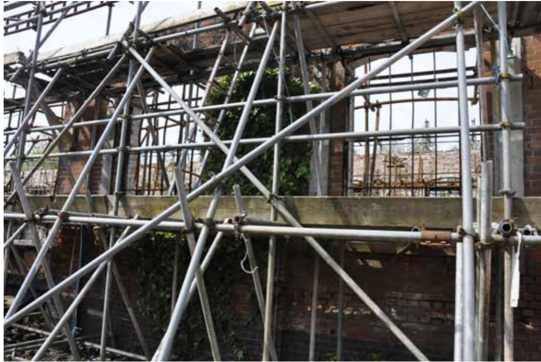
Figure 15: Detail of east elevation showing detail of damaged cast-iron casements (2016)
