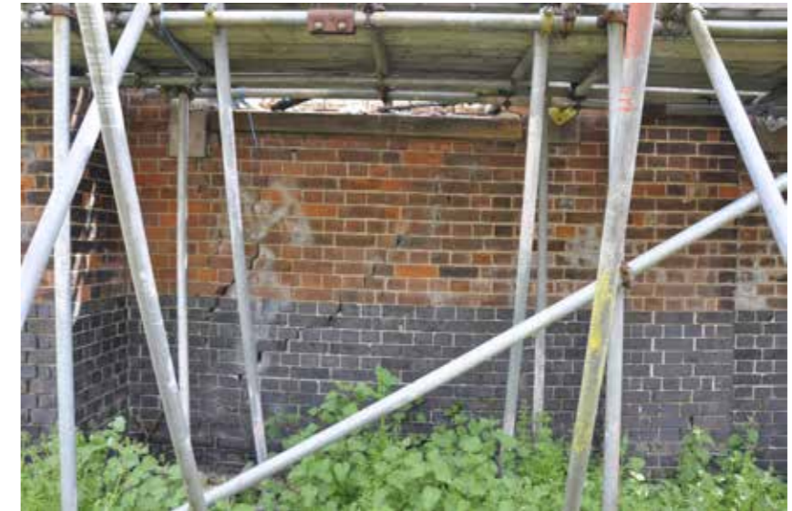
Figure 27: Detail of north-west corner showing subsidence and damaged cast-iron casements on first bay (2016)
