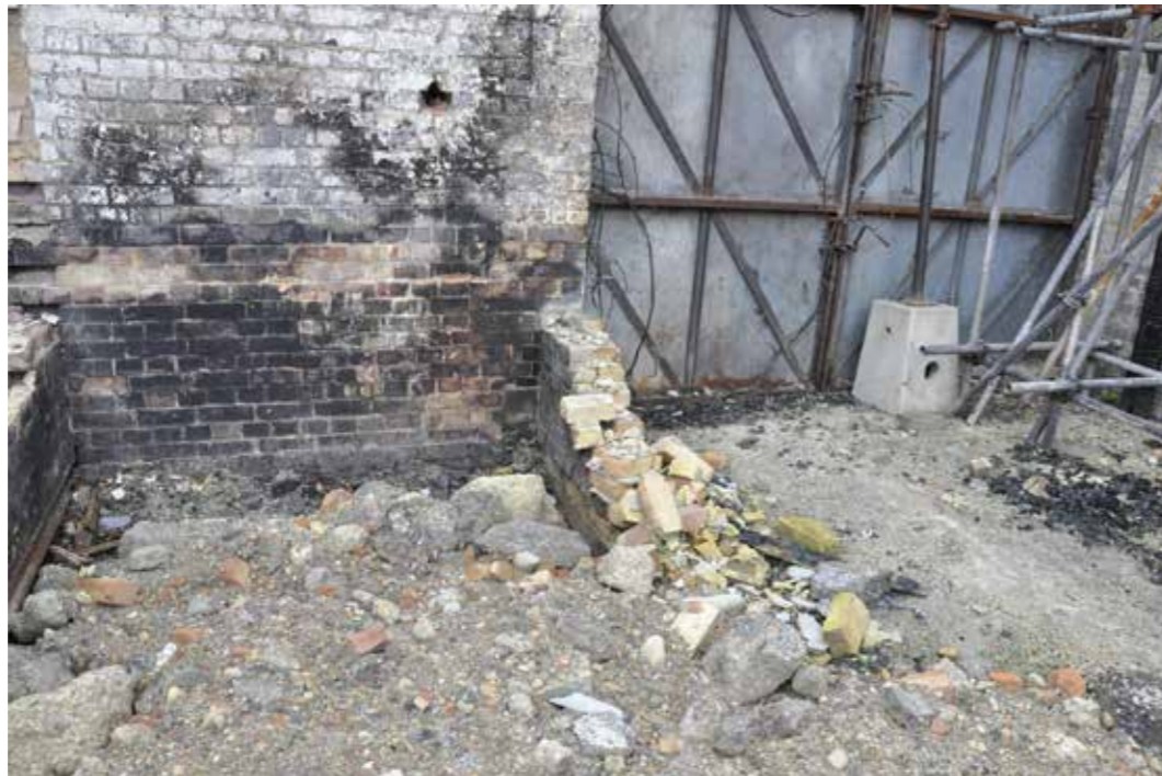
Figure 50: Detail of damaged interior platform structure and steel doors (2016)
