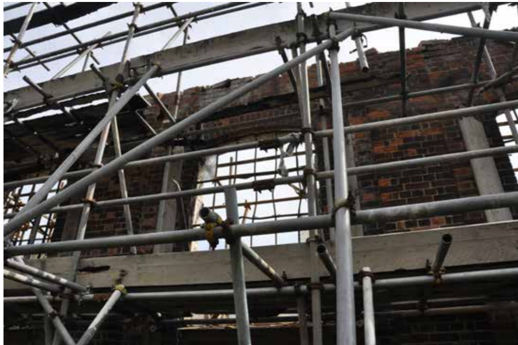
Figure 23: Close-up detail of west elevation showing damaged cast-iron casements and loss of roof (2016)
