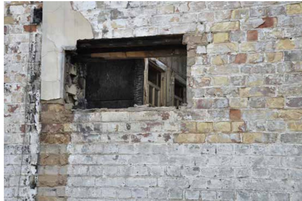
Figure 51: Detail of small office interior showing sash windows as seen from shed (2016)
