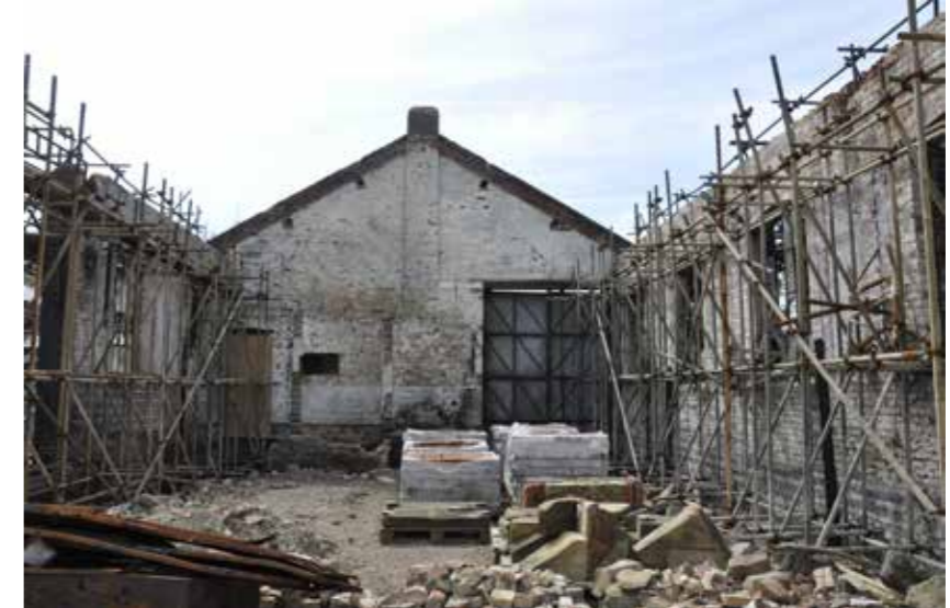
Figure 43: General shot of shed interior showing loss of fixtures and fittings (2016)
