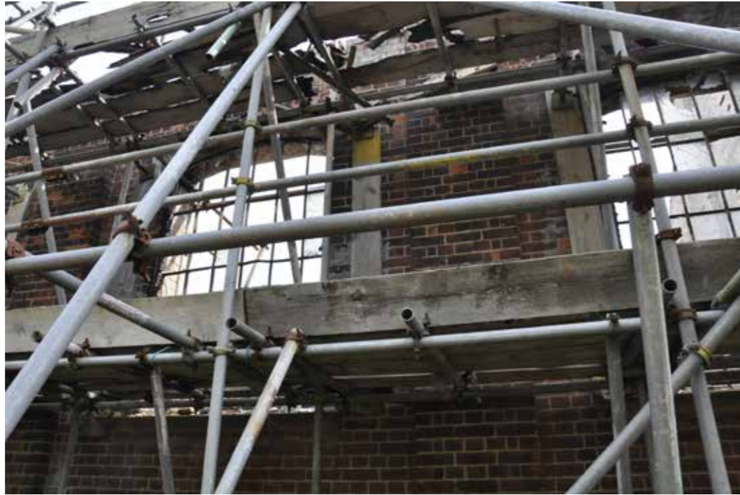
Figure 21: Detail of west elevation showing damage to cast-iron casements on the seventh bay window and the less damaged eighth bay window (2016)
