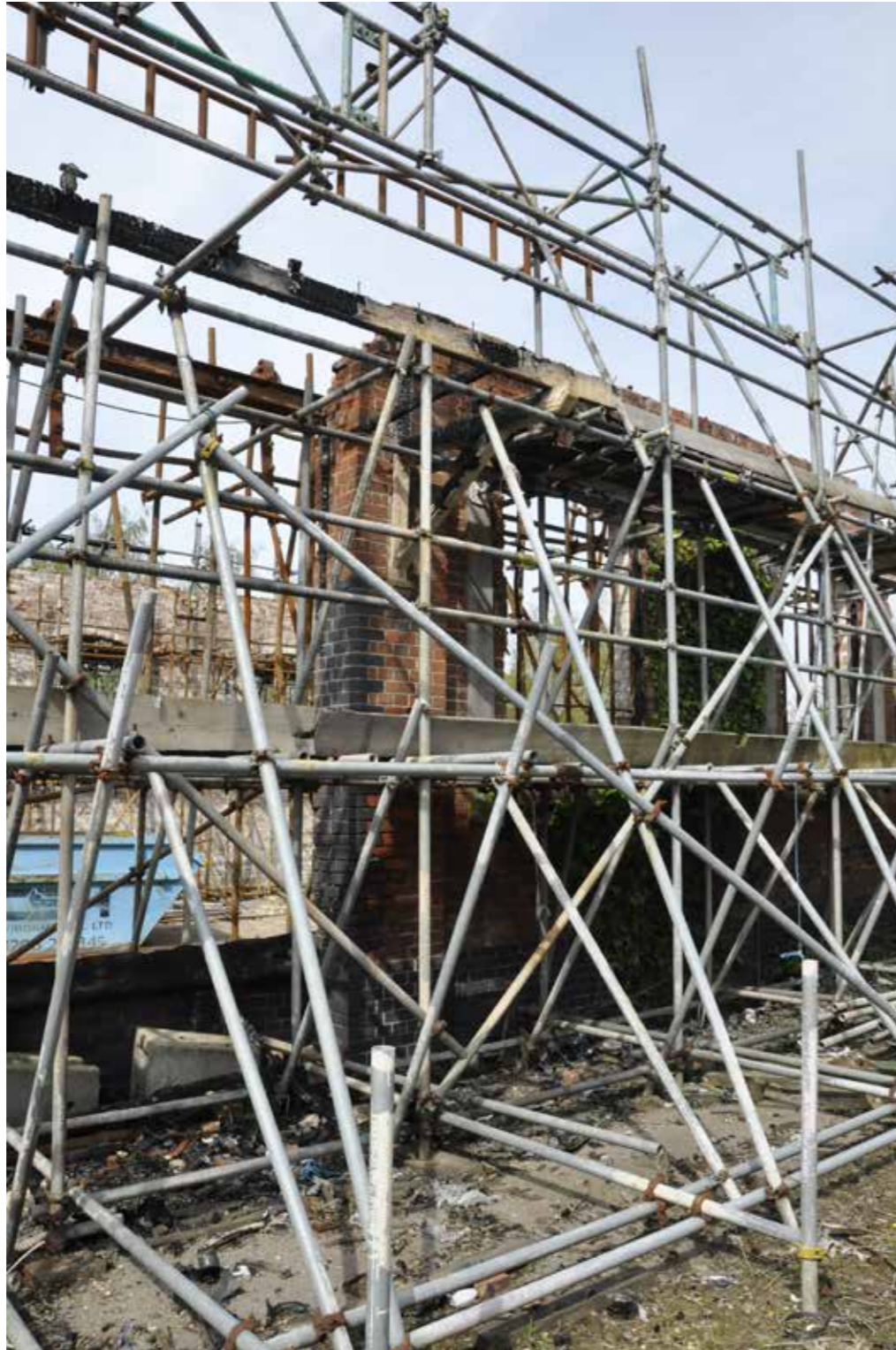
Figure 19: Detail of east elevation showing damage to second lean-to canopy, damage to cast-iron casements and loss of roof (2016)
