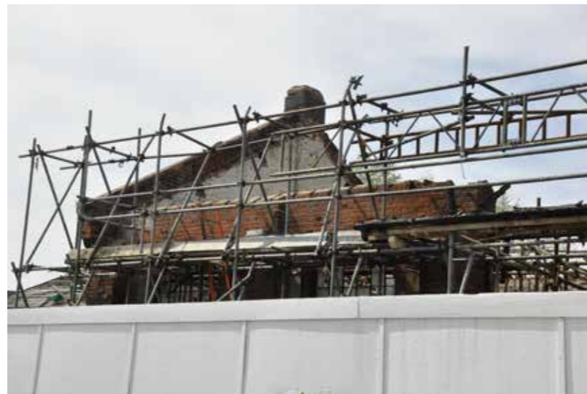
Figure 13: Detail of south elevation seen from the station car park (2016)
